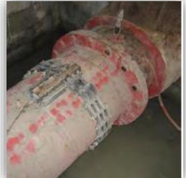
The same installation in 2010. No damage to the HydroFlow despite periods of submersion.
